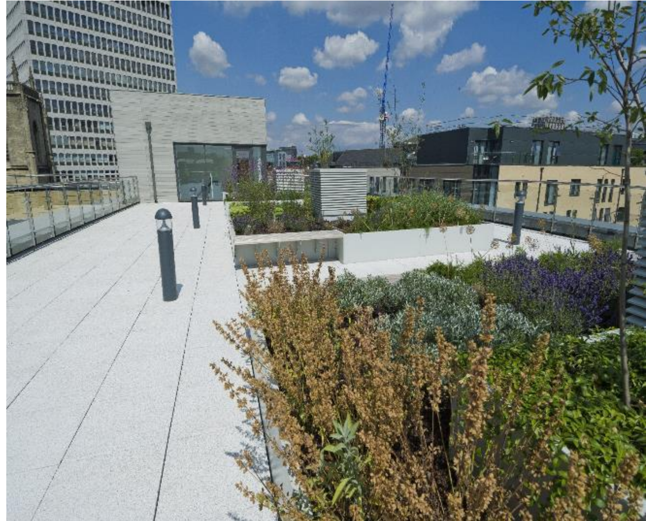
Alumasc Roofing – Derbigum BluRoof – Redcliff Quarter, Bristol
