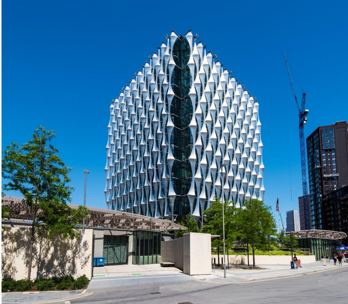
American Embassy, London – Roofing & Water Management
